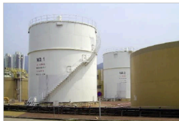
CMHK x ShaTinSTW 5G Remote Inspection
